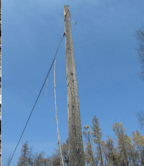
Figure 18: Failed Pole
