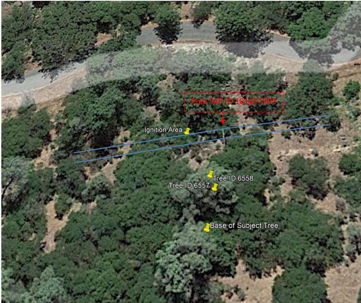
Figure 8: Diagram of the Subject Tree, Tree ID 6557, Tree ID 6558, Ignition Area, and PG&E Facilities. 45 Note that the lines marked in blue show approximate conductor path and continue east and west in both directions.
