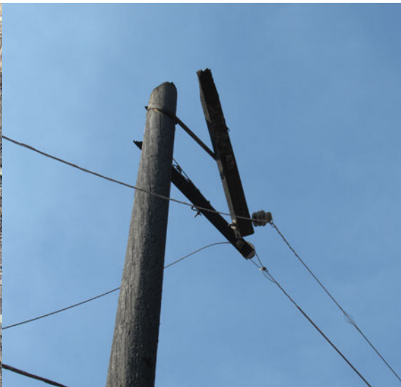
Figure 20: Broken Crossarm
