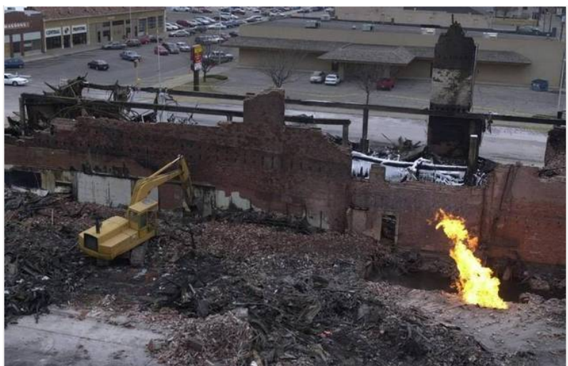
Figure 8. Photo of downtown Hutchinson, KS, after explosion from an underground storage field at Yaggy
