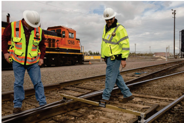
CPUC Track Inspectors taking a track guard check gage measurement in a rail yard.
