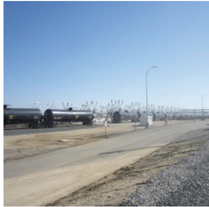
Crude Oil Unit Train at Plains All American Facility in Bakersfield on September 11, 2015
