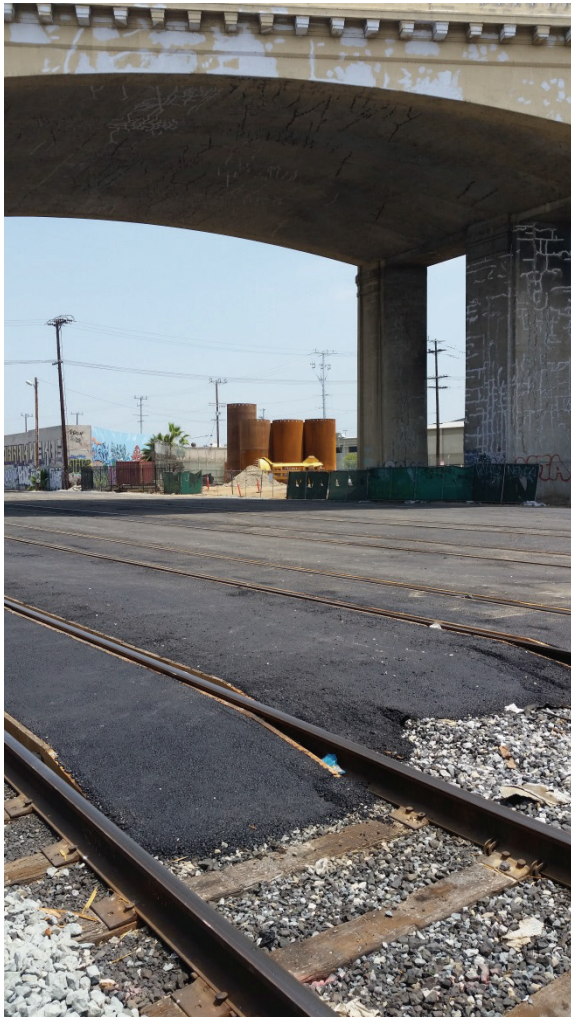
The UPRR 4 th Street Yard and 4 th Street Bridge; hazardous materials tank cars where the pavement was improperly applied.
