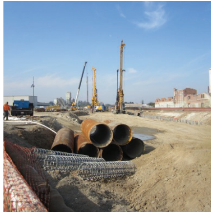
Construction work on the California High Speed Rail Fresno Trench.
