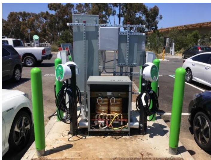
Figure 6. UCSD Site - Installation of 2 dual-headed AeroVironment EVSEs
