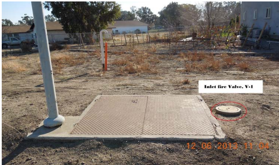
Photo 1- Location of the inlet fire valve located at the first stage
