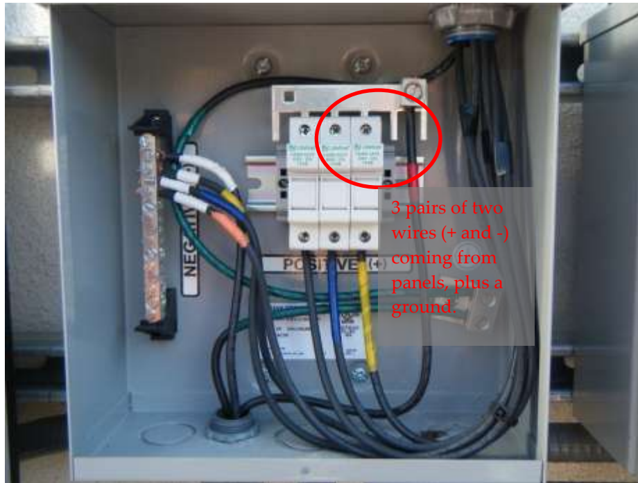
Figure C.2. Typical DC Fuse Box
