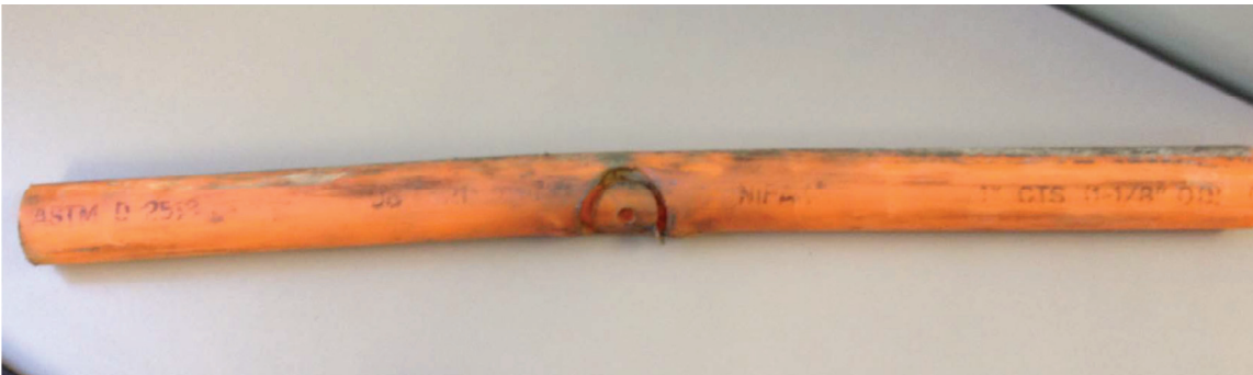
Figure 2. NIPAK TR-418 pipe with welding damage (Data Request #4160 "TR-418.pdf").
