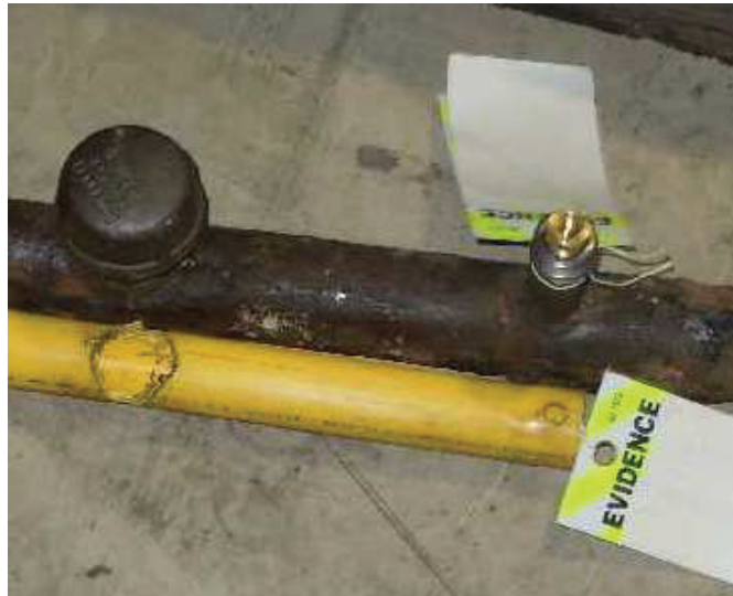
Figure 8: Damaged plastic main insert and steel casing showing two damaged locations.
