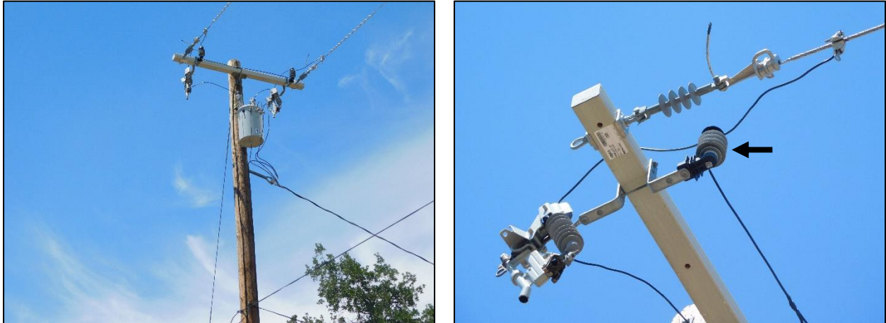
Figure 9: New Pole/New Equipment/Non-Exempt Lightning Arresters
