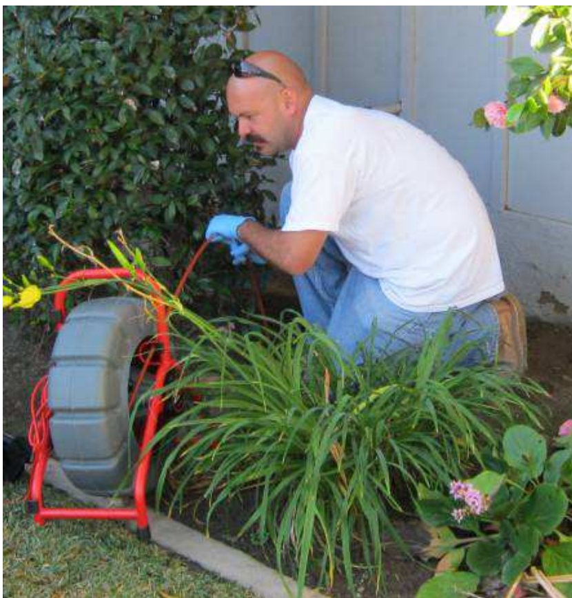
Camera in customer's clean-out
