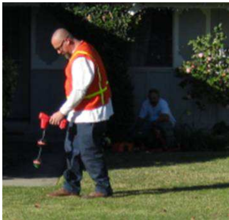
Locating sewer lateral
