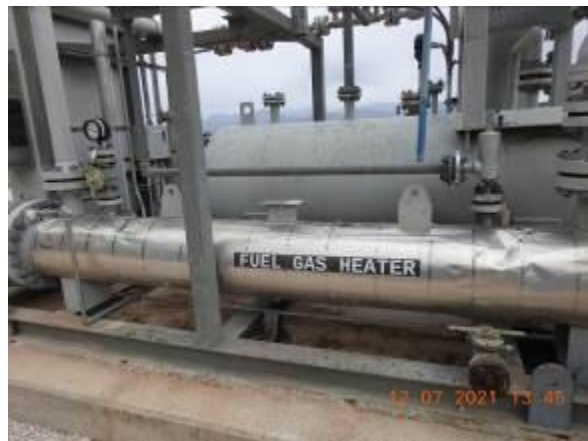
Damaged insulation
