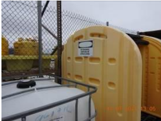
Faded Danger sign in the hazardous waste storage area
