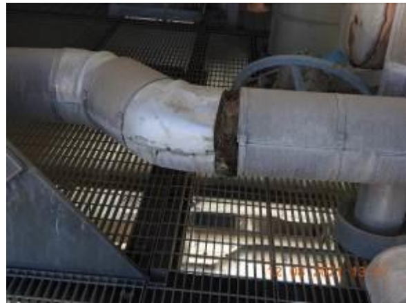
Damaged insulation
