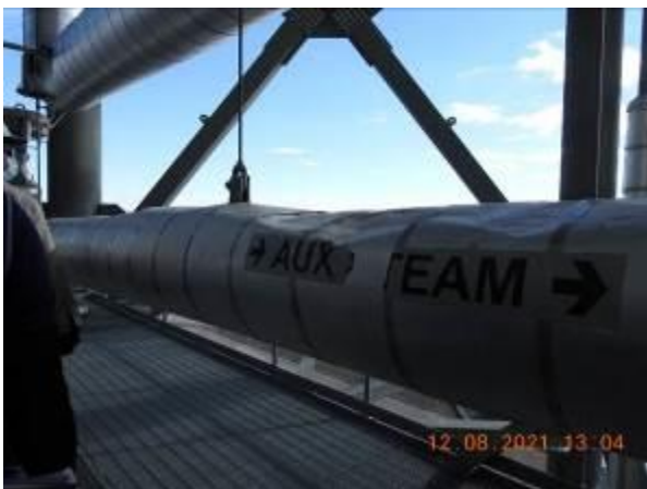
Damaged insulation
