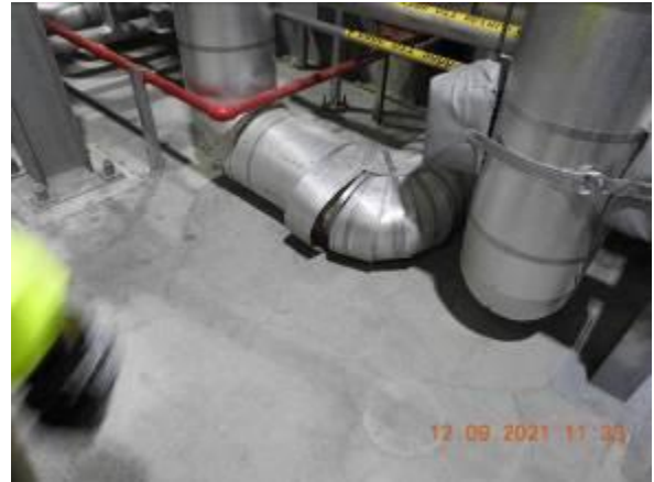
Damaged insulation
