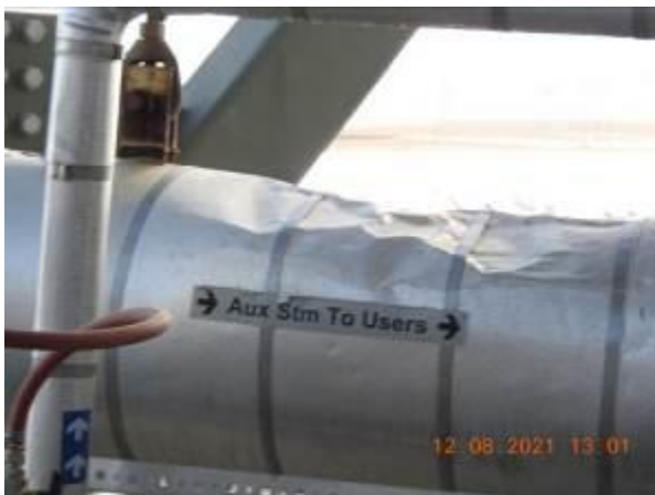
Damaged insulation
