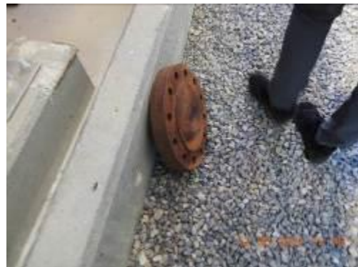
Debris left near the ammonia loading station
