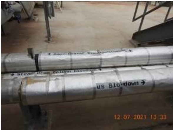
Damaged insulation
