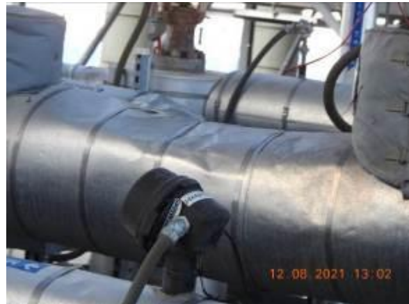
Damaged insulation
