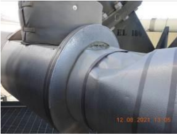
Damaged insulation
