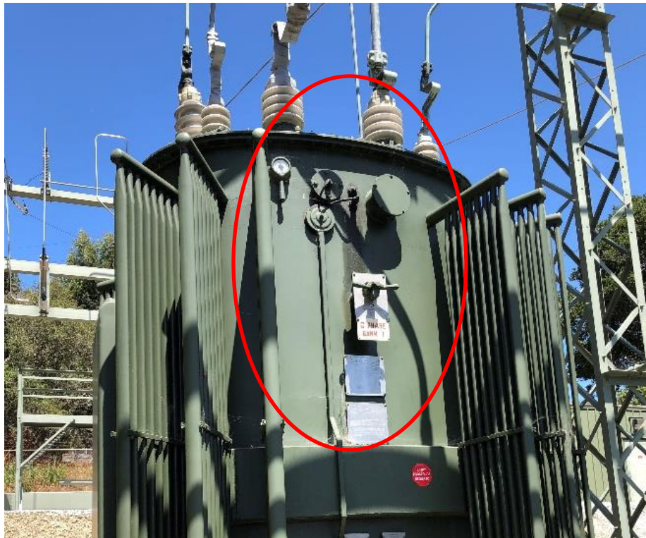
b. Oil leak at the temperature probe of Bank 1C.
