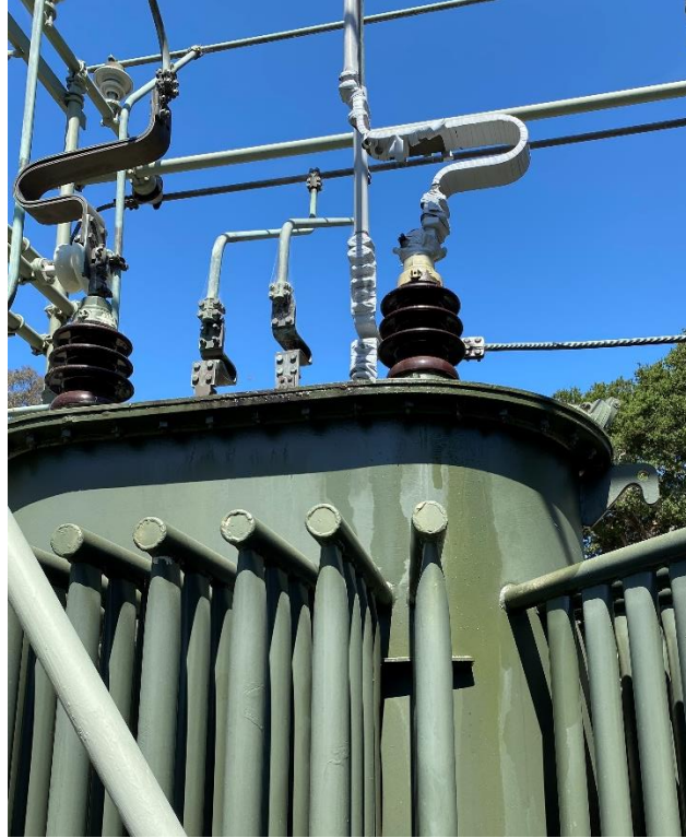
b. Oil leak at the temperature probe of Bank 1C.
