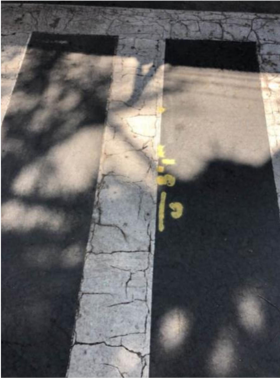
Image 7: Marks in area described on expired USA Ticket #A191060668 believed to be provided by Cable, Pipe and Leak locating employees.
