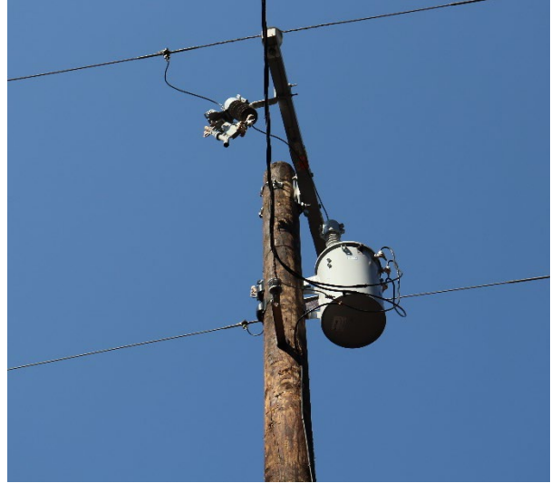
Figure 6: New pole (Pole 1) and transformer
