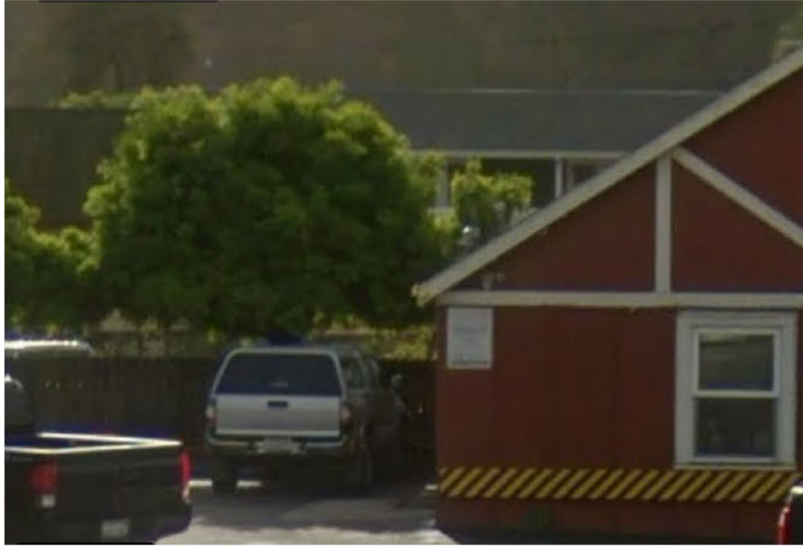
PRIOR TO FIRE – View from Main Street toward 'A Matter of Taste' parking lot
