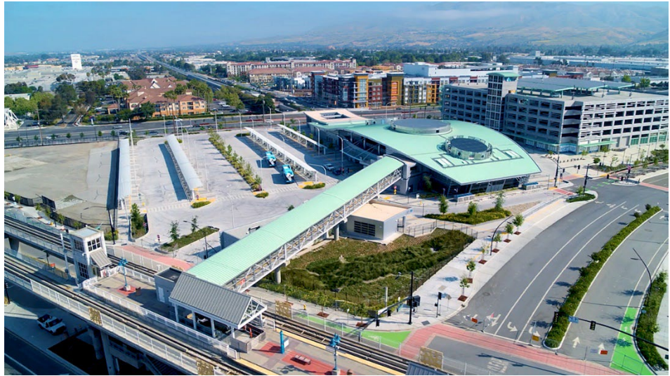
Milpitas Transit Center, connection between BART and VTA Light Rail
