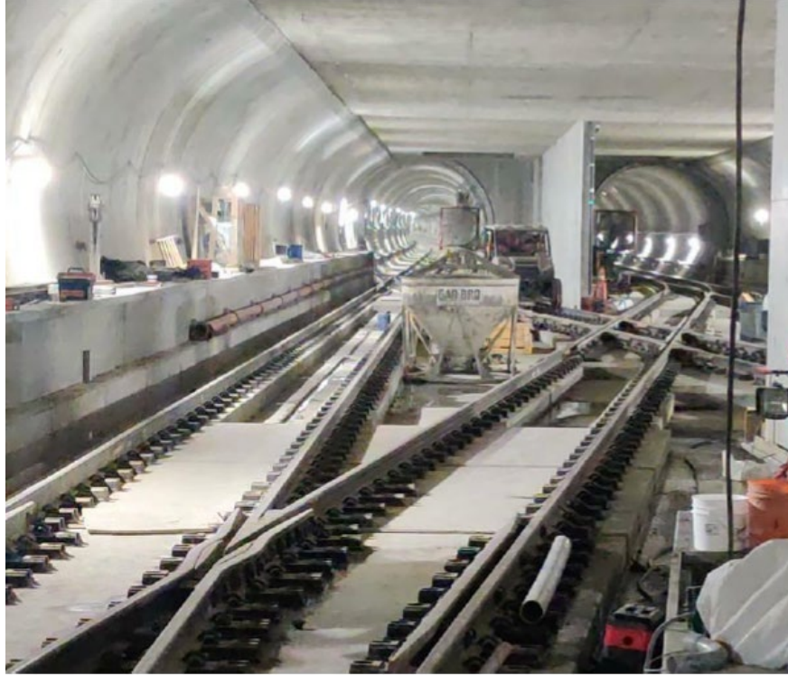
Overview of Crossover Cavern adjacent to Historic Broadway Station
