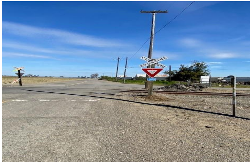
After: Photo received from CFNR manger showing the passive warning device at the Best Ranch Road crossing has been repaired, now properly displaying warning signs. Additionally, the crossbuck sign has been replaced due to faded lettering.
