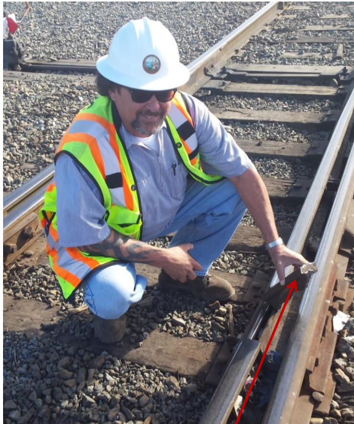
A CPUC inspector holding the broken rail piece
