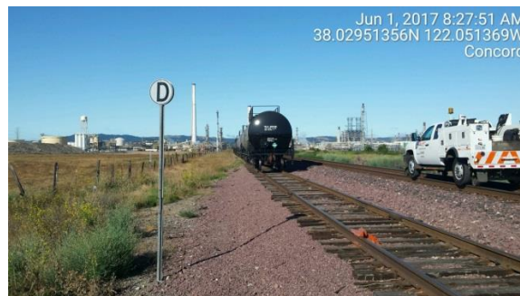
View of the chemical plant track. Tesoro Refinery is on the right and the chemical plant is on the left. The truck is sitting on the BNSF main track between Oakland and Stockton with train speeds of 70 MPH.
