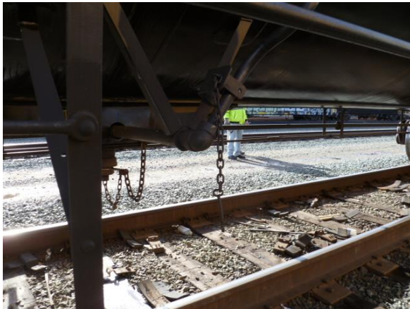
Securement pin found hanging from chain, allowing the valve handle to move to an open position
