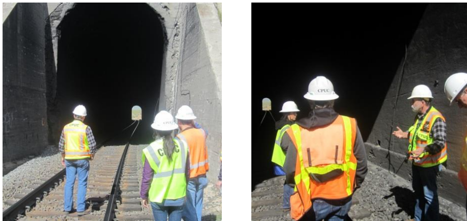
CPUC risk assessment team at a tunnel observation in the Tehachapi Pass area
