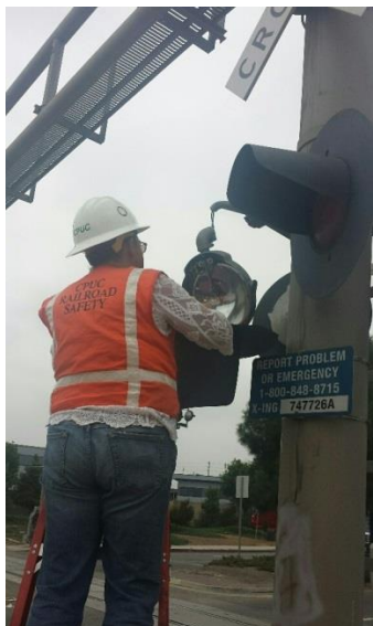
A CPUC Signal & Train Control inspector during an at-grade crossing inspection
