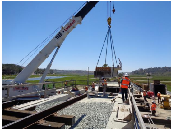
Railroad contractor removing a bridge span
