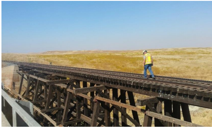
A CPUC track inspector inspecting track over an open deck bridge
