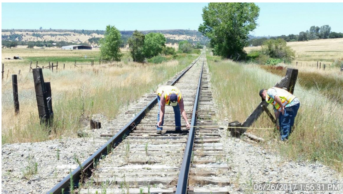
CPUC inspectors measure for side clearance compliance
