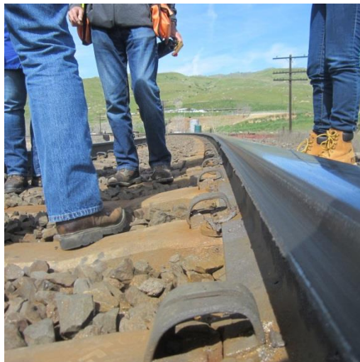
CPUC staff examining worn rail on a curve
