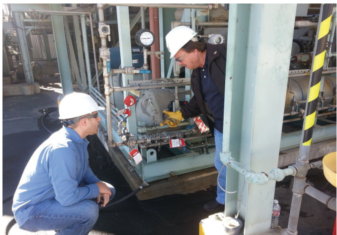
CPUC inspector inspects power plant repairs
