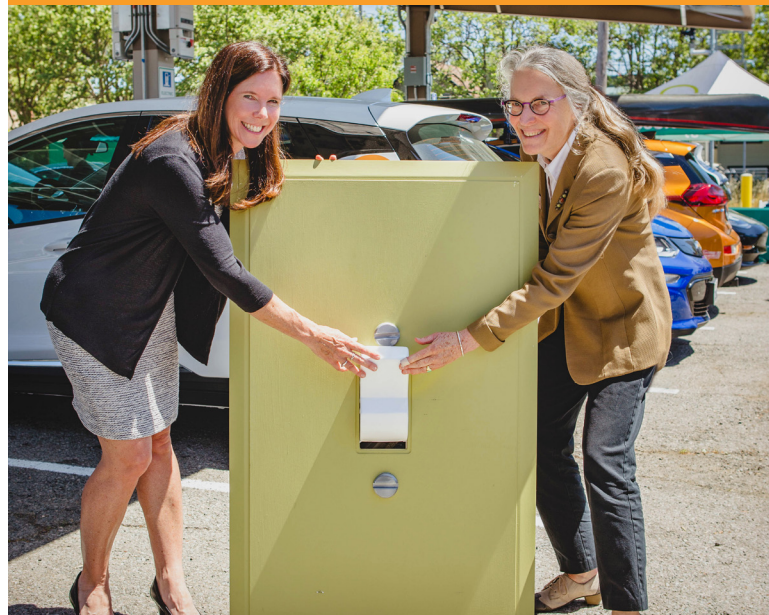
Below: Weisz flips the switch on MCE Solar Charge in San Rafael with former MCE Board Chair, Kate Sears.
