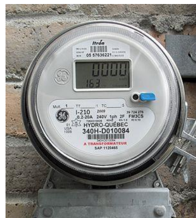
Figure 3 Example of Solid-State Electric Utility Meter
