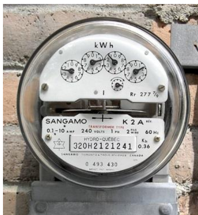
Figure 2 Example of Electromechanical Electric Utility Meter
