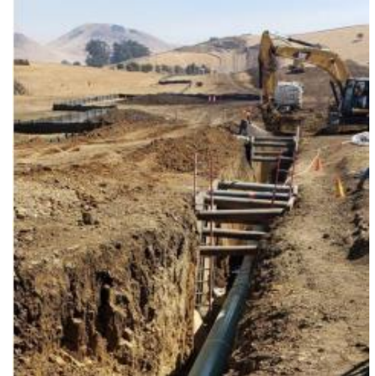
Pipeline Replacement for Green Valley Fault in Fairfield
