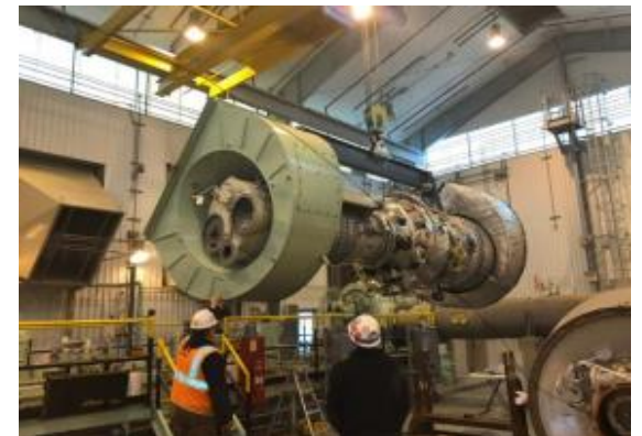
Delevan Compressor Station Turbine Exchange
